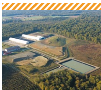
Disposal facility for VLL (very low level) waste located in the industrial centre for collection, storage and disposal (Cires) in the Aube département.
