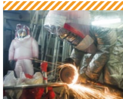
Specialists equipped with dedicated suits in order to deal with radioactive waste contaminated with plutonium.
