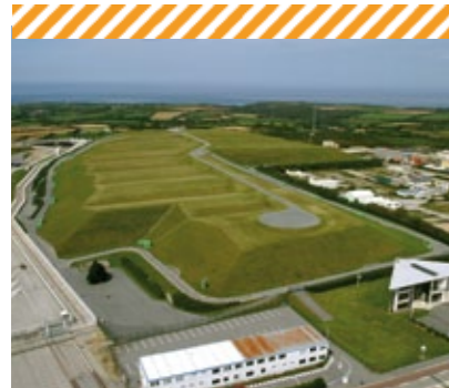
Aerial view of the Manche repository (CSM) at Digulleville.
