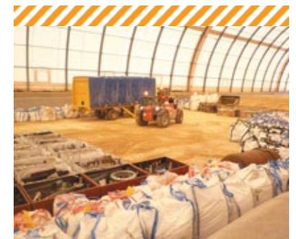
Emplacement of VLL waste in a disposal cell excavated at a depth of several metres in clayey rock.
