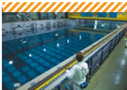
After being used in the reactor, the spent fuels are stored in pools filled with water, so that they can cool down. The height of water provides protection against the radiation they emit.
