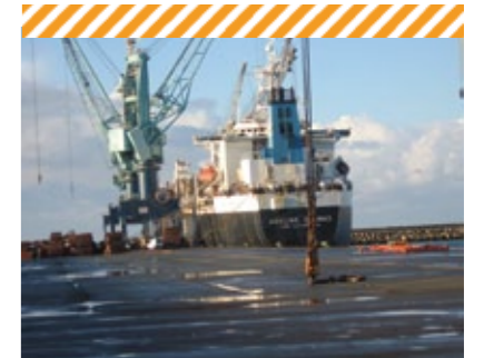
Port of La Pallice in La Rochelle (17) where production residues (VLL type waste) from the Solvay plant (formerly Rhodia) were used as backfill in the construction of the port.
