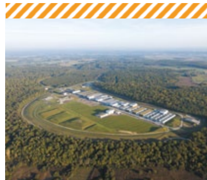
Surface repository for LLW/ILW (low/intermediate level waste) at Soullaines-Dhuys (in the Aube département).
